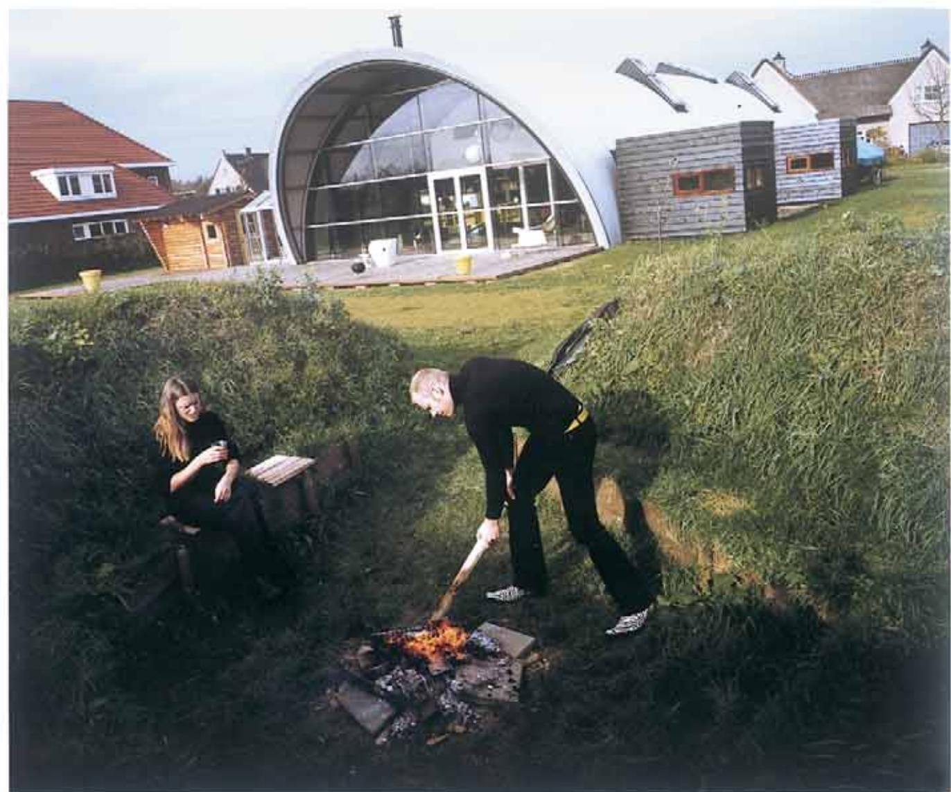
In the enclosure between the interior and exterior walls of this corrugated steel construction, almost 1.1 miles of piping brings water in for heating/refrigeration. A glass wall on the south side is an additional, "passive" heater during the winter.
